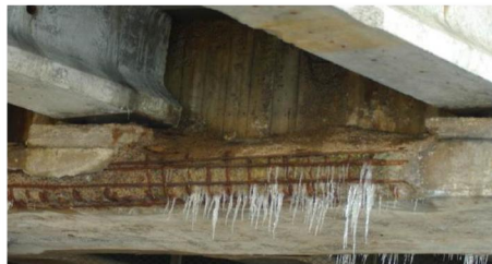
Freeze-thaw damage
