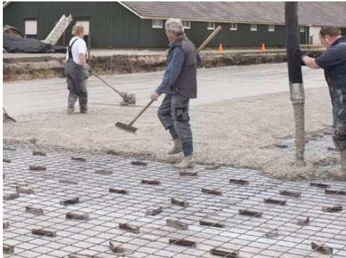
Acid-resistant concrete floor in a milk factory in Gorinchem, 400 m 3 geopolymer concrete (C53/C60) from Van Nieuwpoort Betonmortel was casted, 2015
