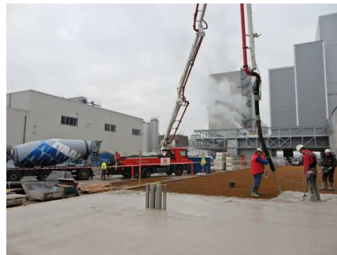
Acid-resistant concrete floor in a milk factory in Gorinchem, 400 m 3 geopolymer concrete (C53/C60) from Van Nieuwpoort Betonmortel was casted, 2015
