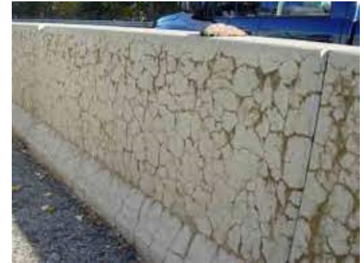
Free expansion: crack formation in all directions
