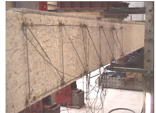
Restrained expansion: crack formation only in X-direction
