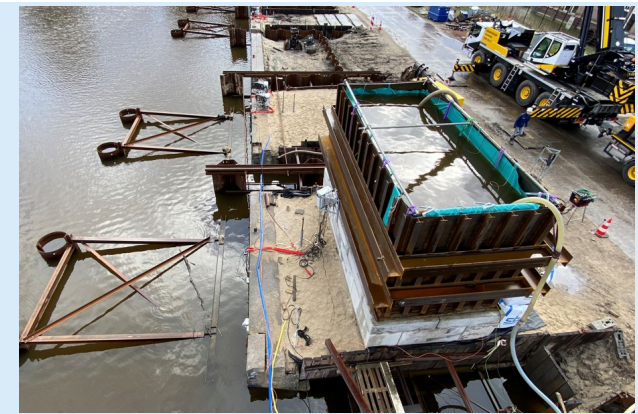
Urban quay wall (2022)
