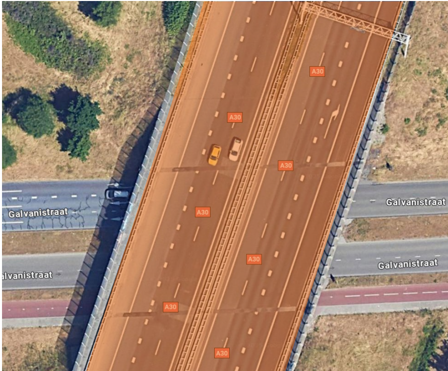
Skewed viaduct bridge KW4 “Frankeneng” in A30 (Ede)
